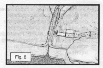
You are finished installing the Sumpto-Sump Drain Connector. Now it is time to install two Stainless Steel Joining Clips.
