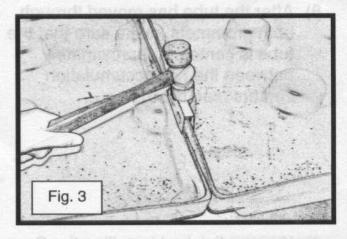
Make sure that the clip is all the way down and flush with the top edge of the accumulation centers (see fig. 4)
